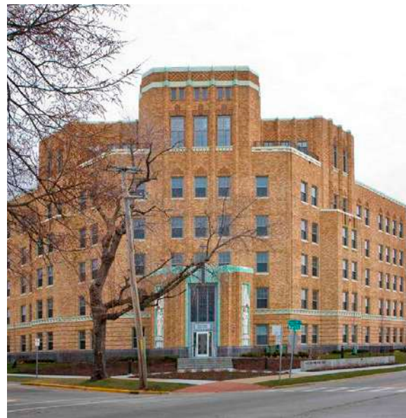
The historic St Charles Hospital in Aurora IL was restored and converted to senior apartments using a variety of incentives.
