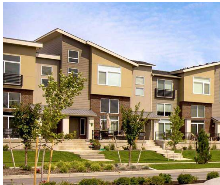
Development in Kendall Yards that utilized the City's MFTE incentive to effectuate redevelopment.
