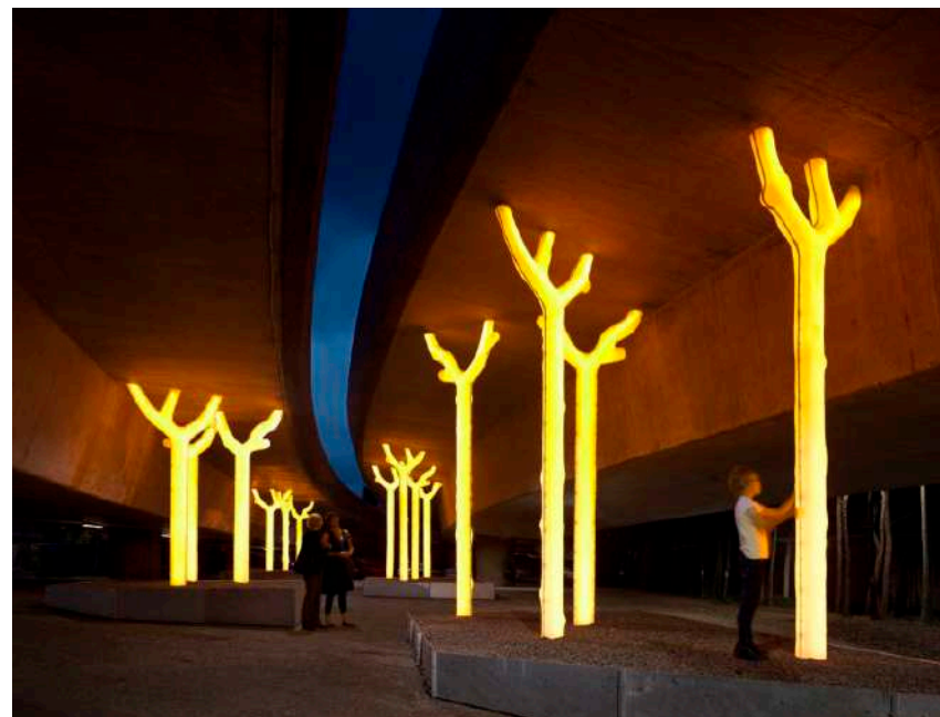
Warren Langley's ASPIRE light sculptures create a safer, more pedestrian friendly beneath a highway in Prymont, NSW, Australia
