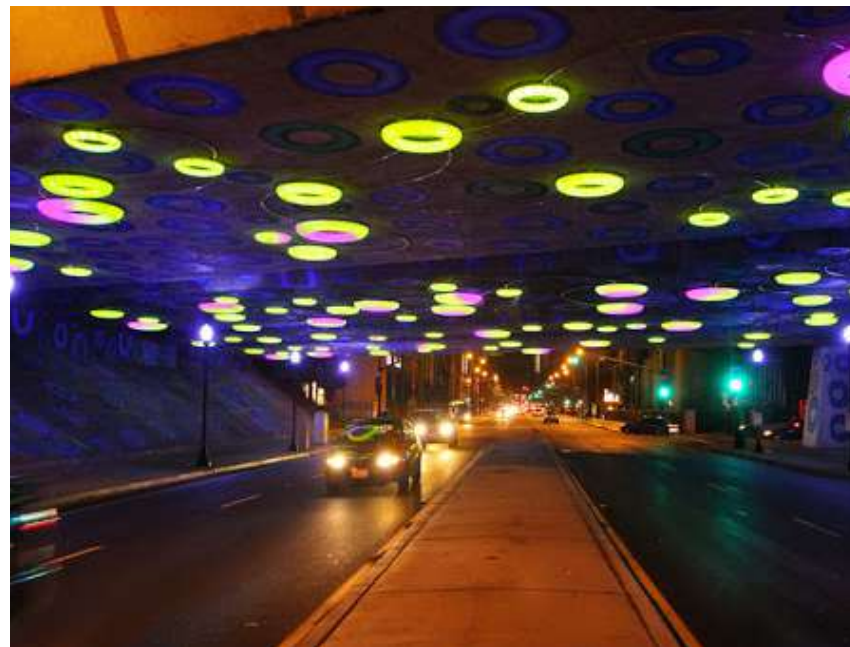
A highway underpass in San Jose, CA redesigned to create a safer pedestrian experience with art by Dan Corson that includes painted surfaces, circular lights LED lighting coordinated with pedestrian scale light fixtures along the sidewalk.
