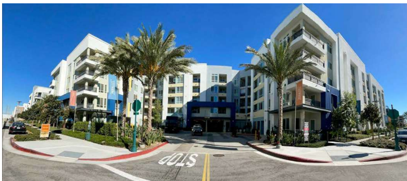
The City of Anaheim, CA created over 1,000 middle-income housing units by waiving property taxes on new apartments in Downtown Anaheim and the City's Platinum Triangle
